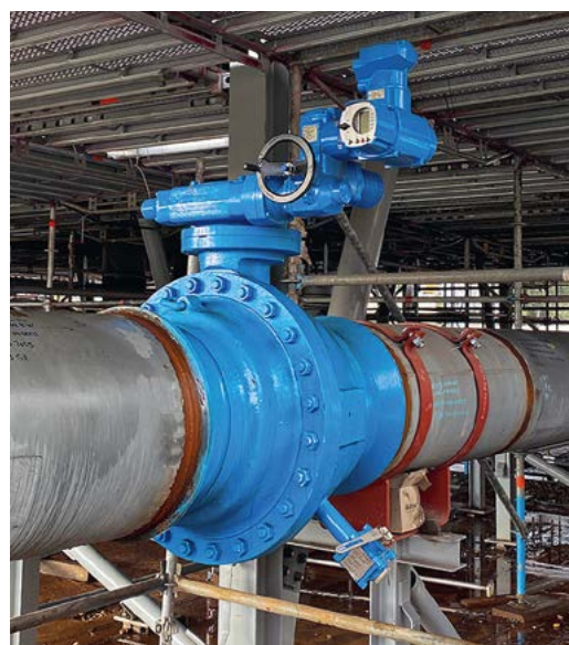
In total, 2,000 Ballostar ball valves have been installed at the CHP plant in Hamburg, Germany.
