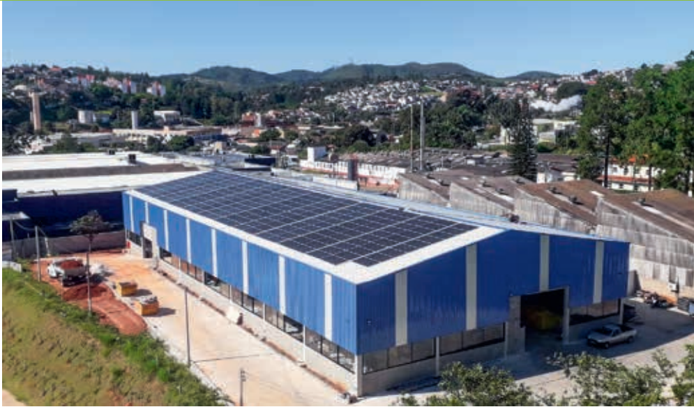
The photovoltaic panels at KLINGER Brazil.
