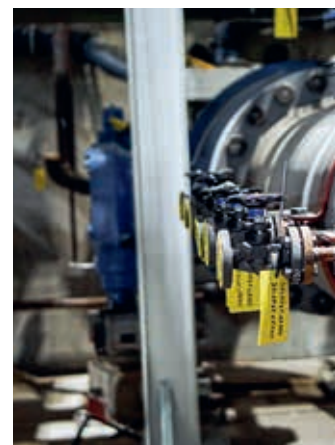
The KLINGER KVN piston valve in its smallest size, DN15, provides venting and draining of pipework.
