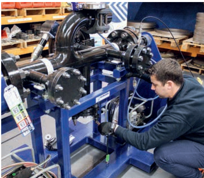
Scott Whelan bolts a flange.
