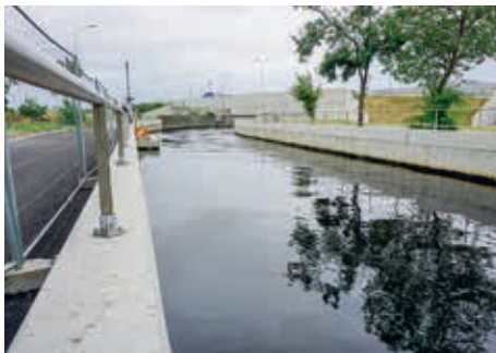
The wastewater comes from Vienna’s adjacent main wastewater treatment plant.
