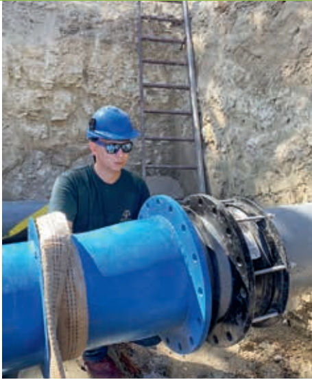
Perfect alignment was key in this delicate project.
