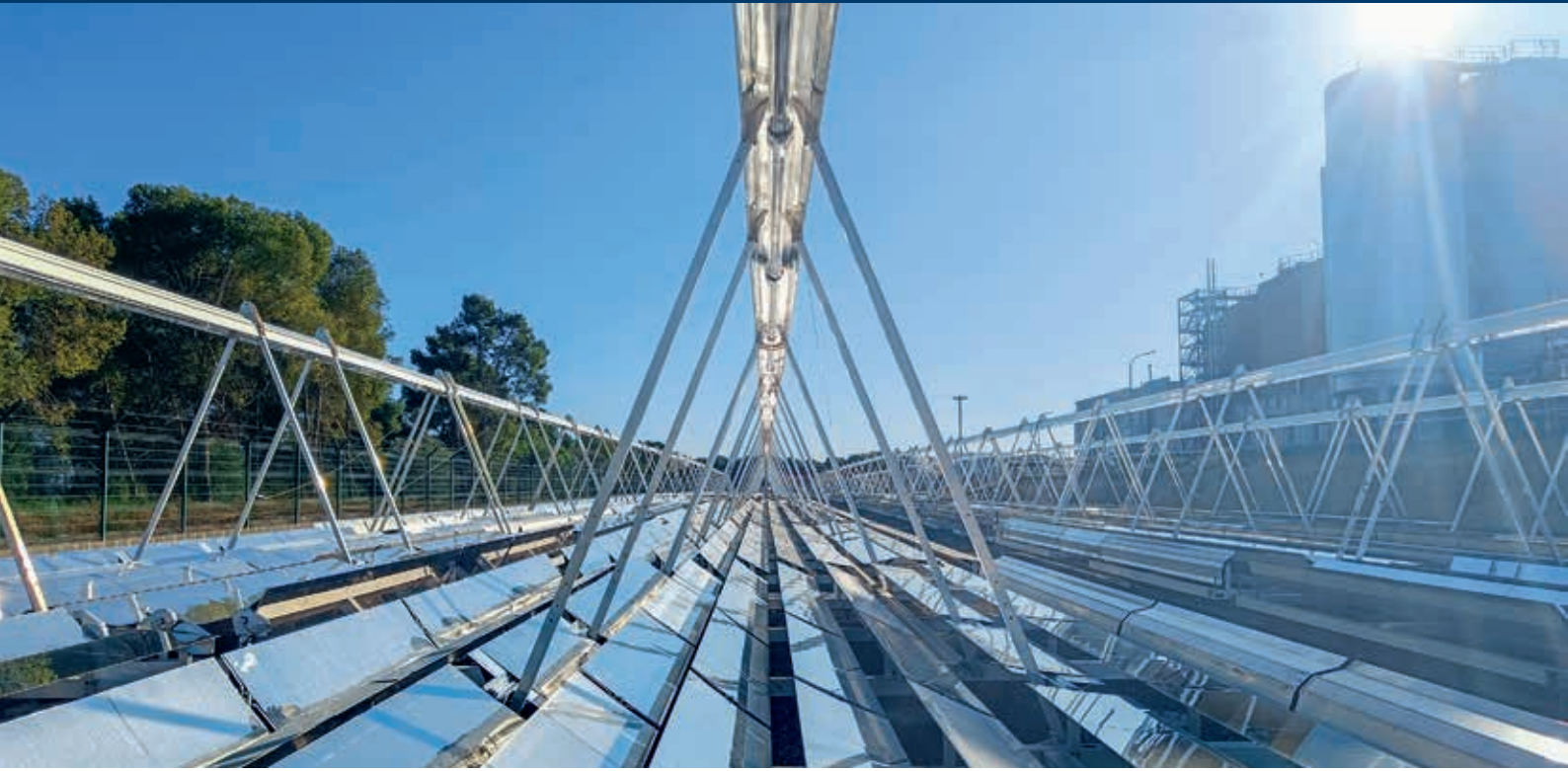
Europe's largest solar steam production plant produces an energy peak of 3.5 megawatts thermal.
